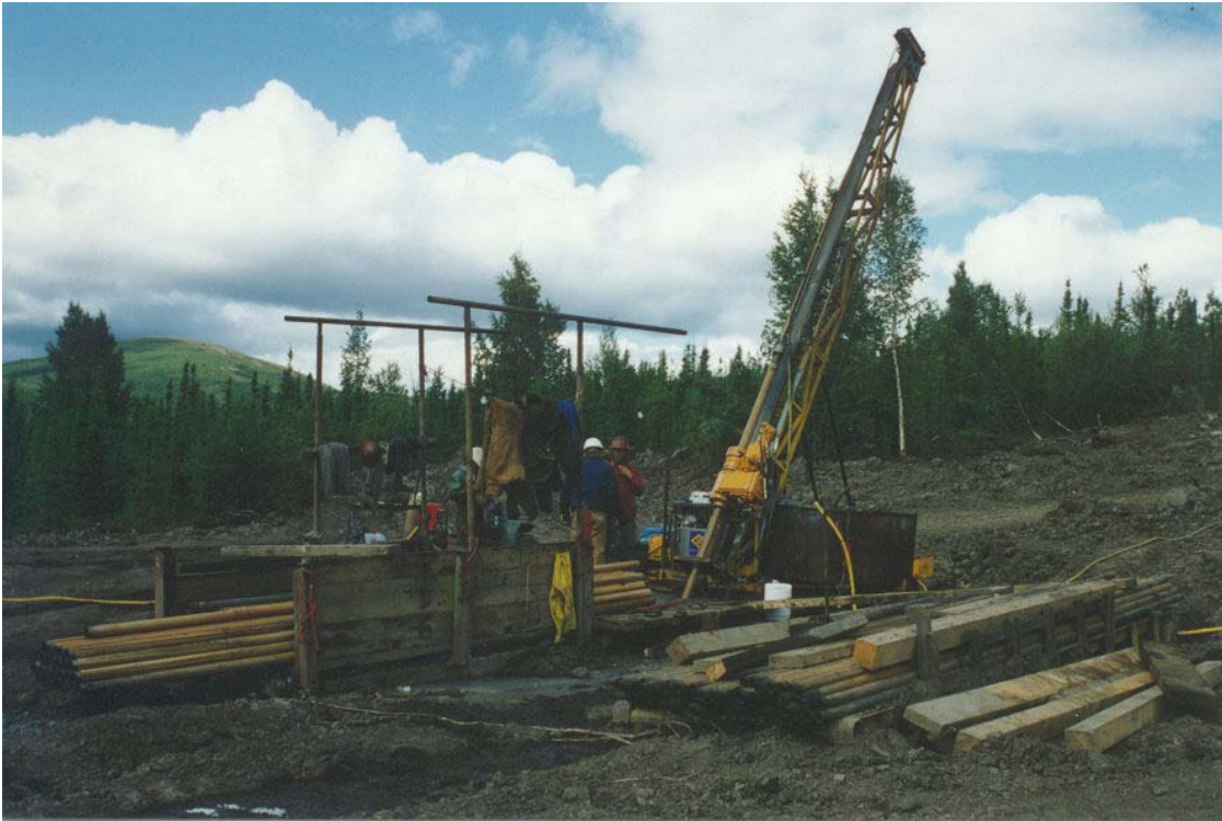
Figure 1 CS 1000 Core Drill Rig
